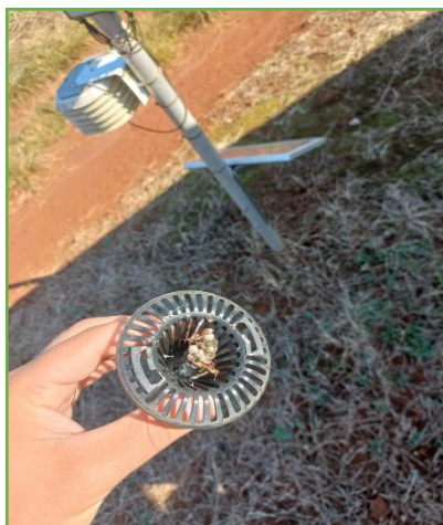
Blocked Rain Gauge. No rain can pour through to the rain tipper resulting in NO rain measurement
